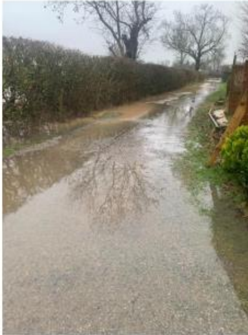
Photograph One- Flooding damage
